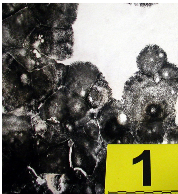
Figure 4 Colonies of Stachybotrys chartarum , the so-called “toxic mold”, developed on a vertical plastered wall affected by rising damp.
